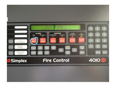
The panel shown is from the Halstead of Holden and it is very obvious where to acknowledge. Once the alarm has been acknowledged, you then can silence and reset as needed.
