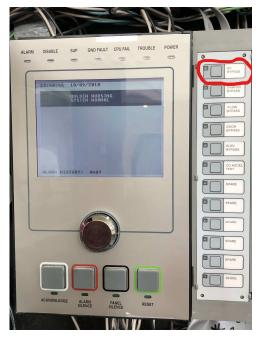
The newer school panels also have this same function if necessary. As for Halstead, to the left of the panel in the previous picture, there is a button marked "city disconnect". This will turn off the alarm system from reporting out to central station, so it should never be left on.
