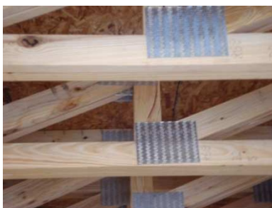
Reserve Interior Roof
